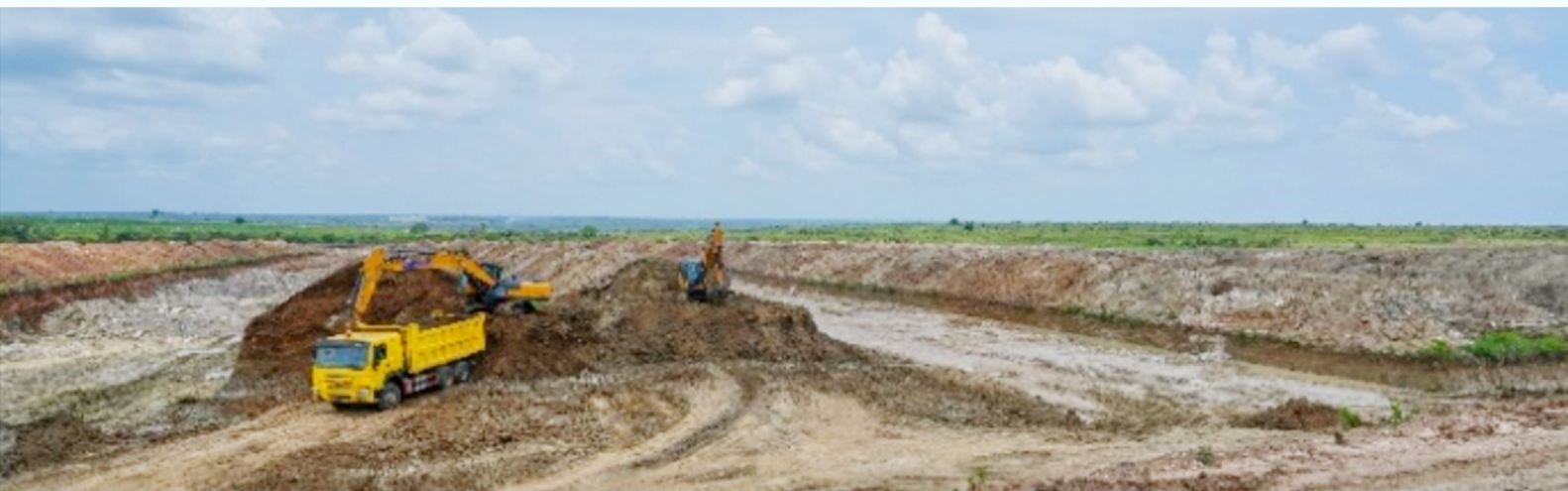
Construction of a new dam
